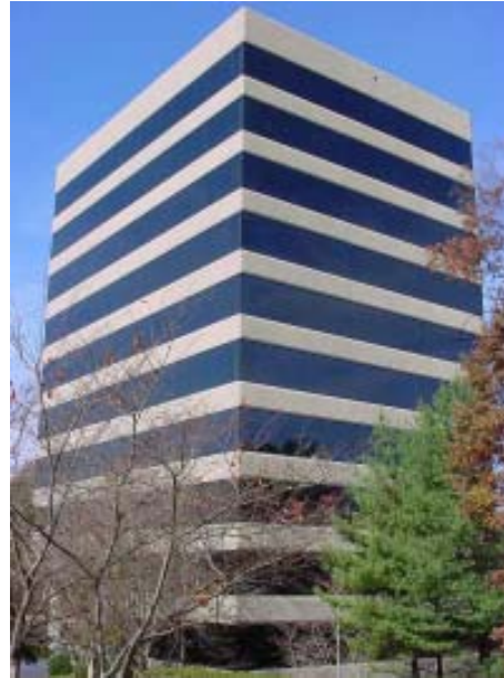
SouthStar Funding Headquarters Atlanta, GA
